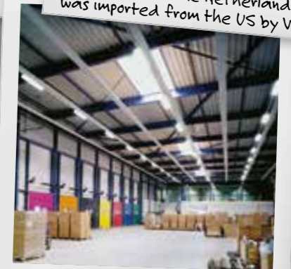
1995 - Line lighting standard equipped with 7 x 2.5 mm 2 flat cable.
