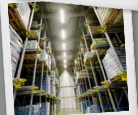
2012 - Narrow-beam LED line lighting with more than 35% savings compared to T5.
